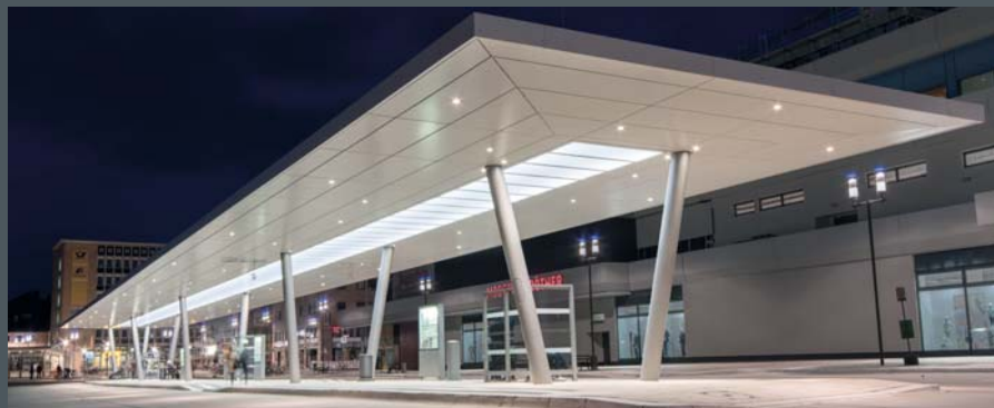
Central bus station, Hildesheim/Germany Lighting design: Studio DL, Hildesheim
